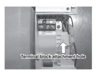
2. Attach terminal block ① using screw ② in the direction shown in the figure.
